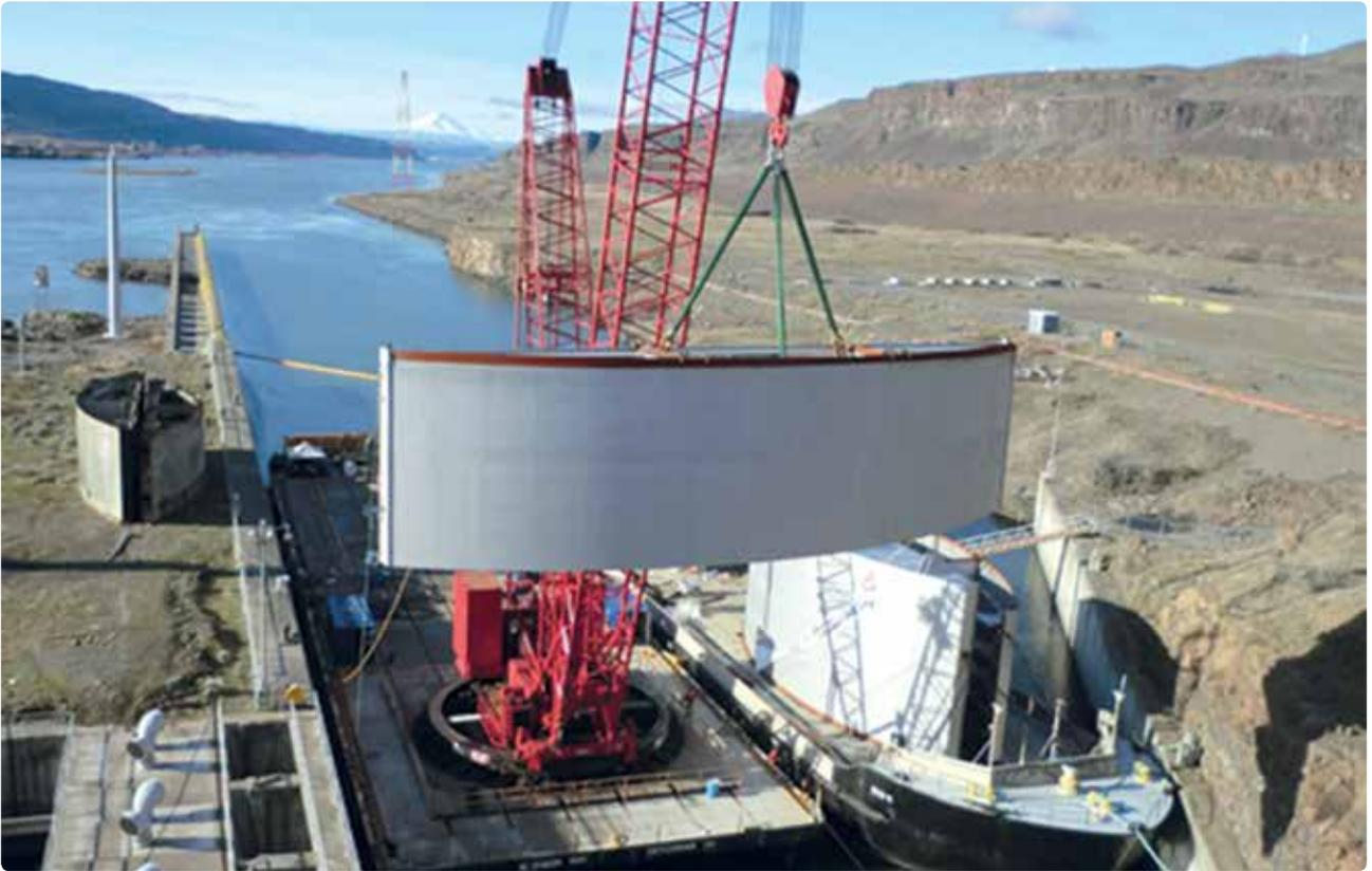
Twin-Path® slings lift a 275 tonne floodgate.
